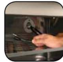
Throughwall Access Port
